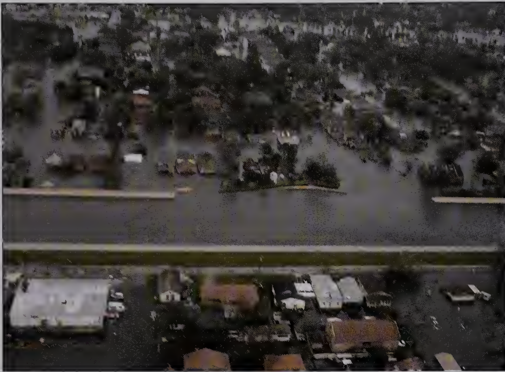
Breached floodwall, New Orleans Marty Bahamonde photo
